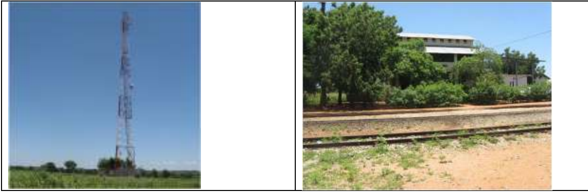
Figures 13a & b are showing the telephone mast and railway station, respectively, in study sites in Dodoma.
