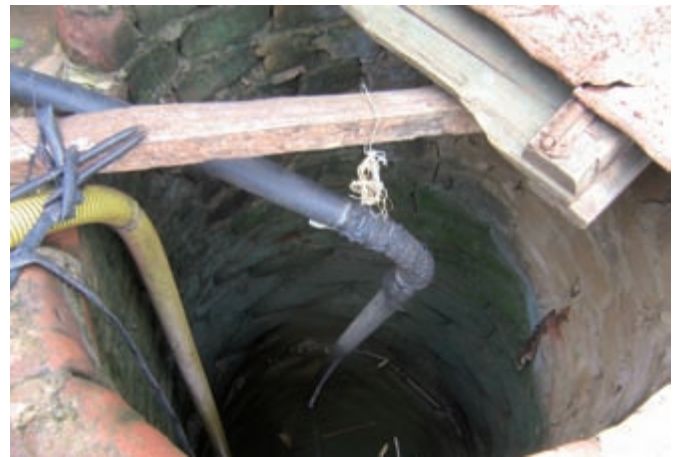
Figure 3: A manual well with motorised pumps as a smallholder AWM in use in Mwebeshi watershed
