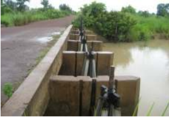
Figure 9. Water regulating structure developed by the LRDP project in Northern Region.
