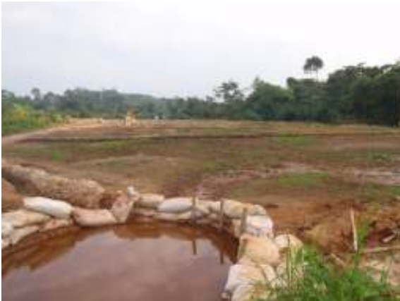
Figure 10. Dyke constructed at one of DIITRPA project sites.
