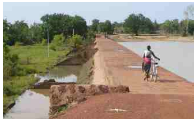
Figure 1: Traversing the reservoir barrier
