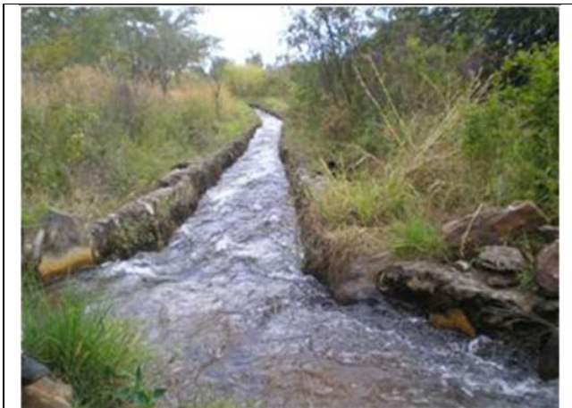
Photo 2. A typical river diversion in Mpika District.
