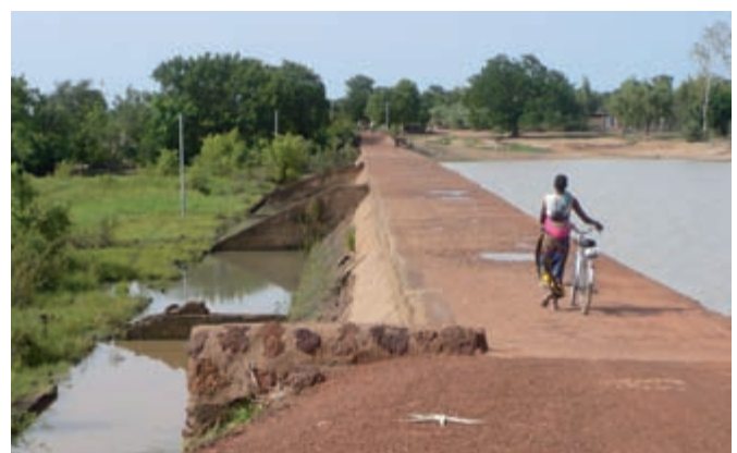
Figure 1: Traversing the reservoir barrier
